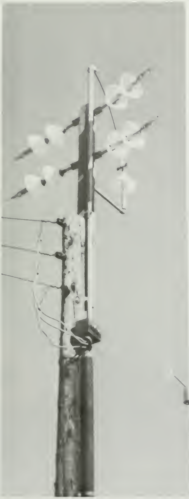
Figure 12. Emission Power Line and Special Insulators Used With Electrical Discharge Method of Cloud Seeding
